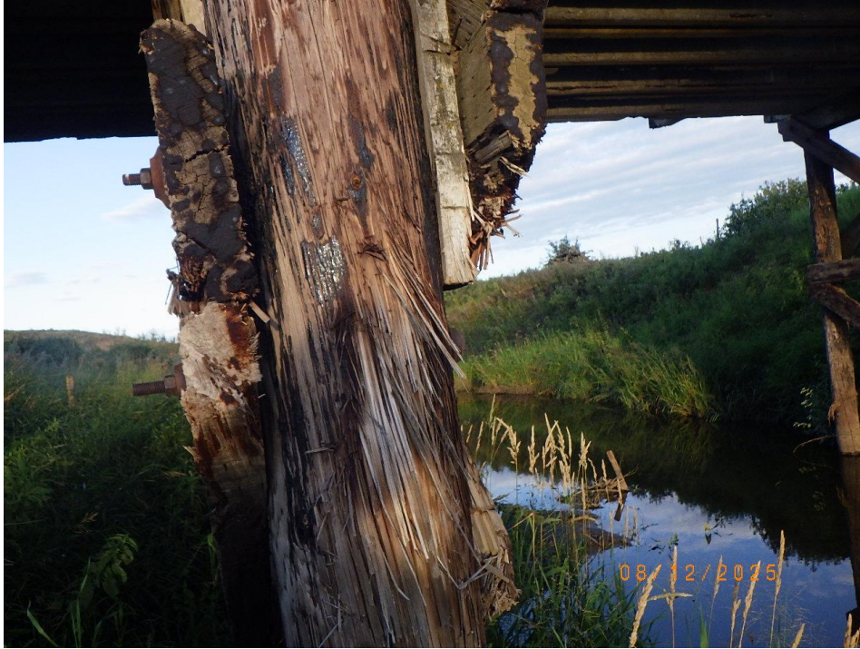
Lead pier pile damaged by drift or ice flows
