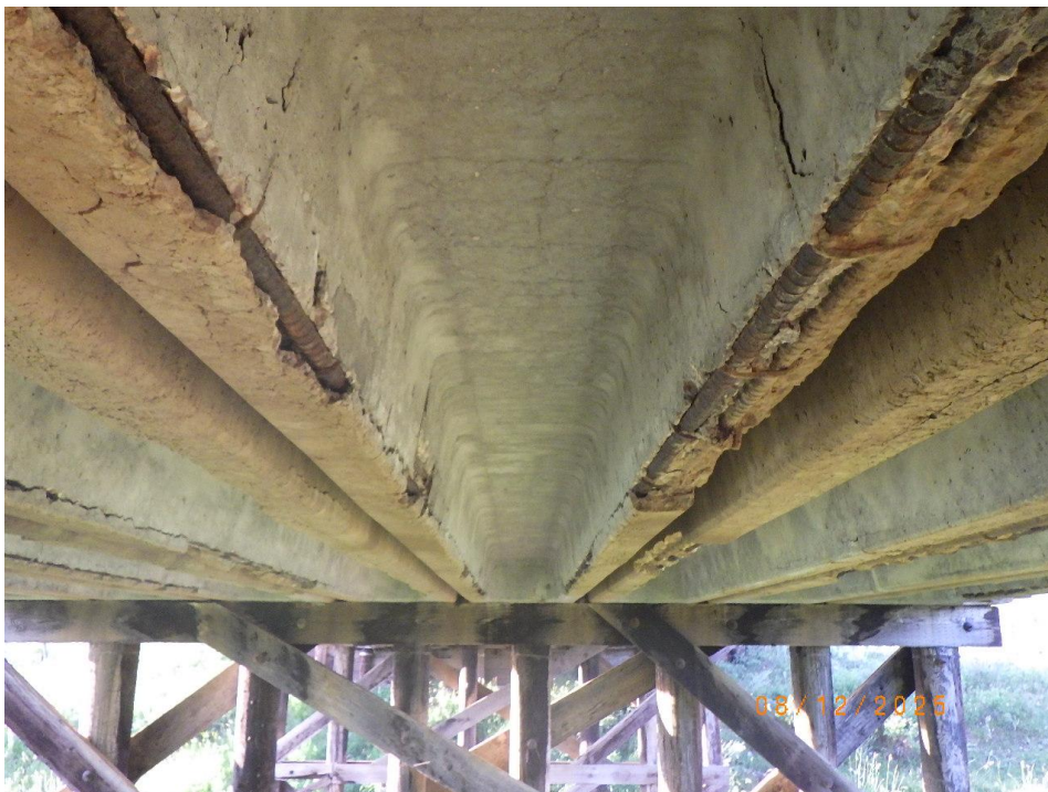
Typical girder spalling due to low cover on stirrups
