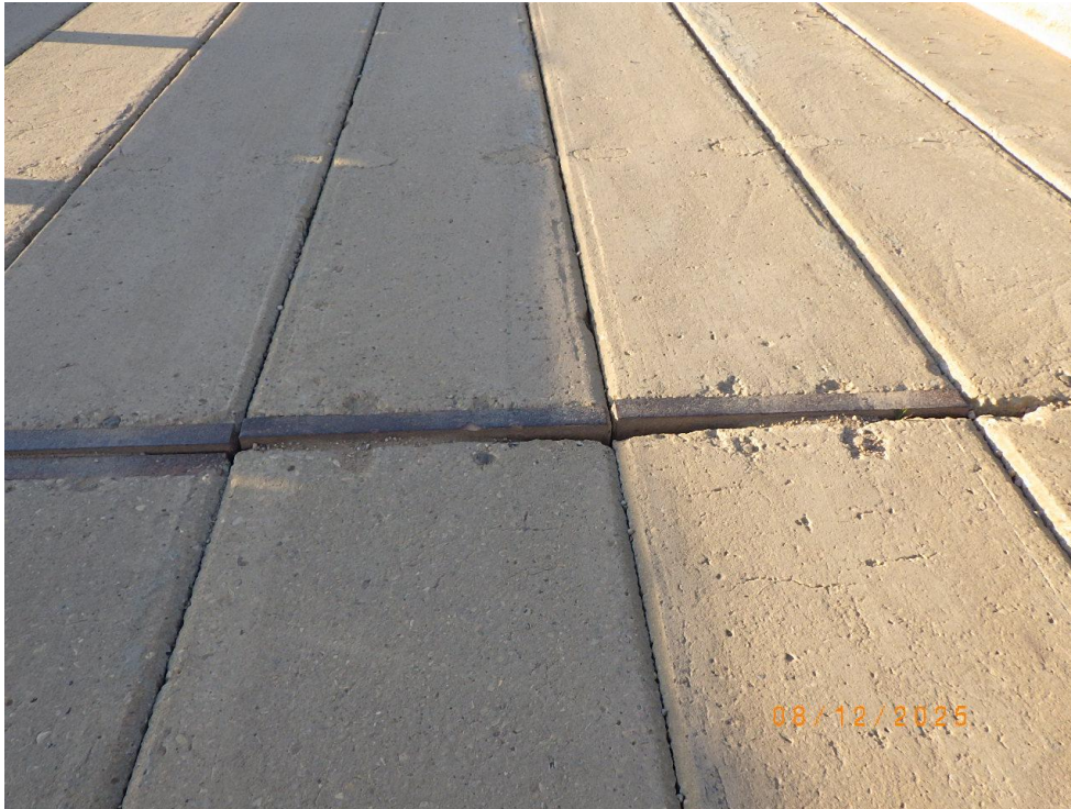
Vertical displacement of the girders at pier 2.
