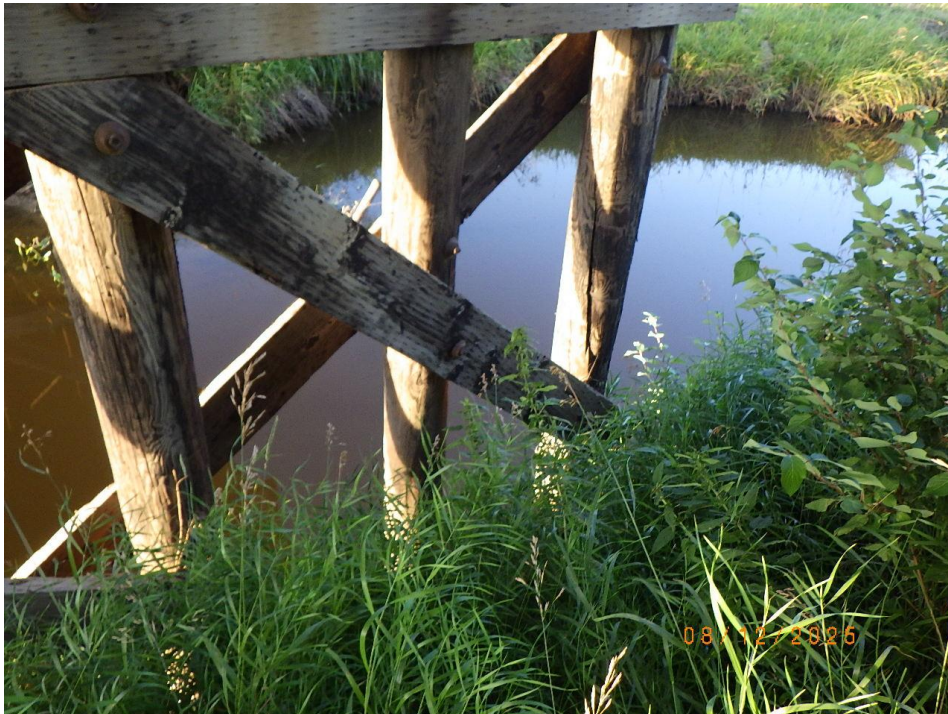
Suspect cracked pile (to be confirmed)
