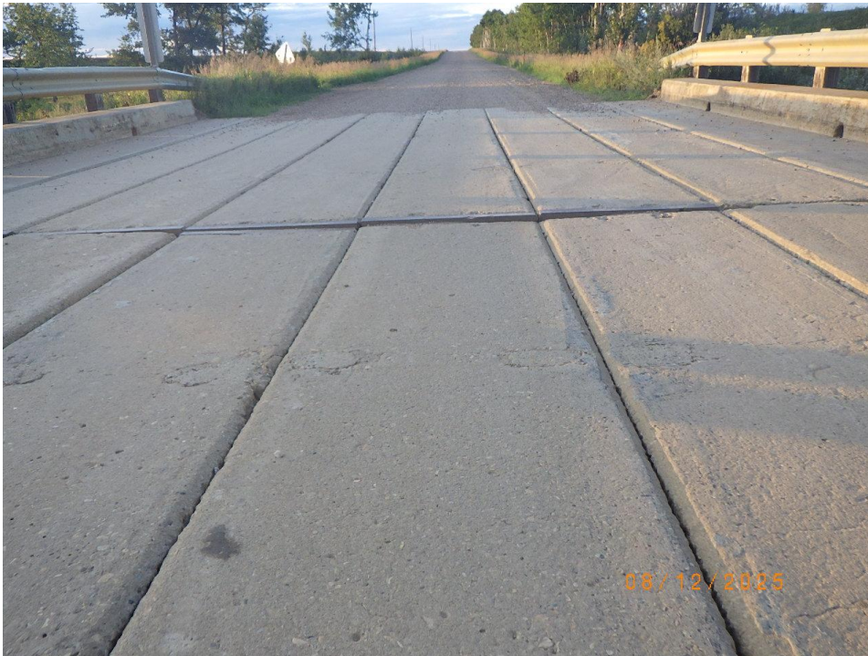
Another view of the displacement at pier 2.
