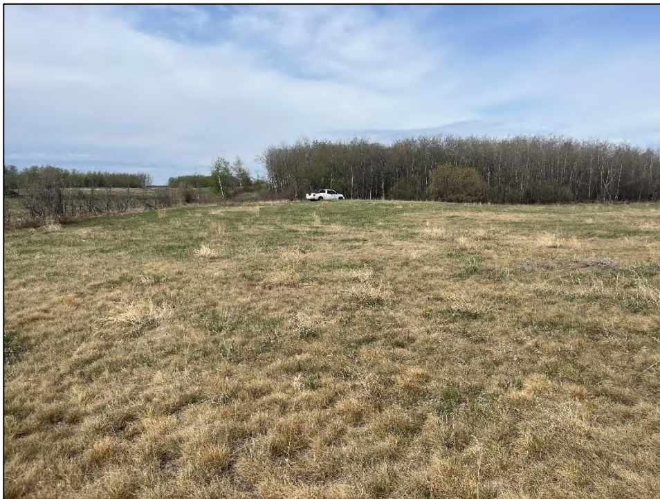
Photo 2. Looking west across site.
