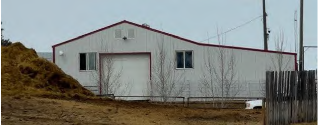
Shop addition without permit approval
