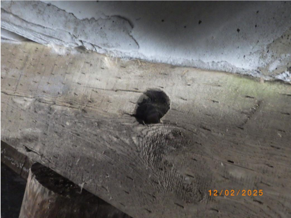
Tieback bolt pulled into crushing cap
