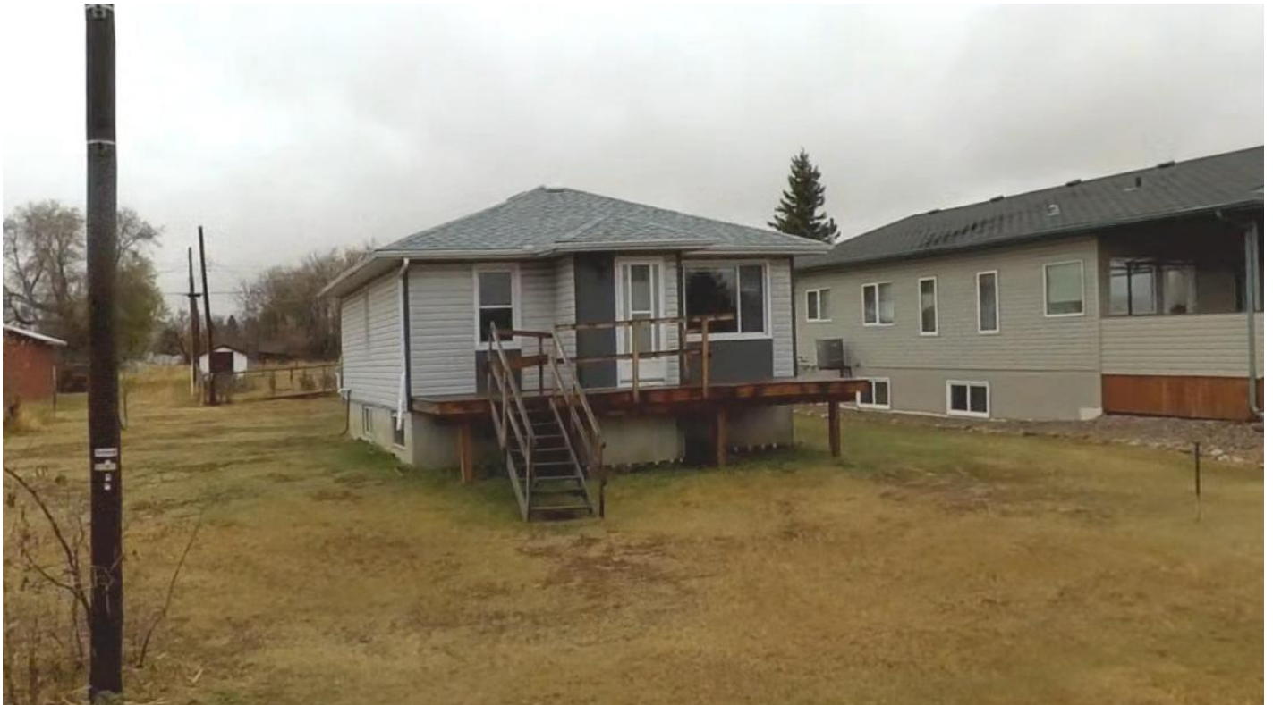
Lot 6A, Block 9 – Dwelling Not Yet Complete
