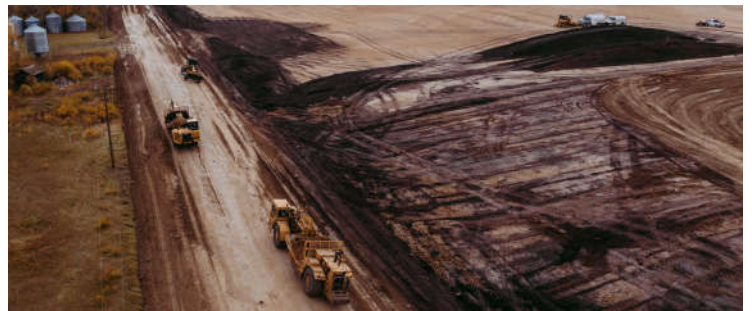
Road grade improvements on Rge Rd 143
