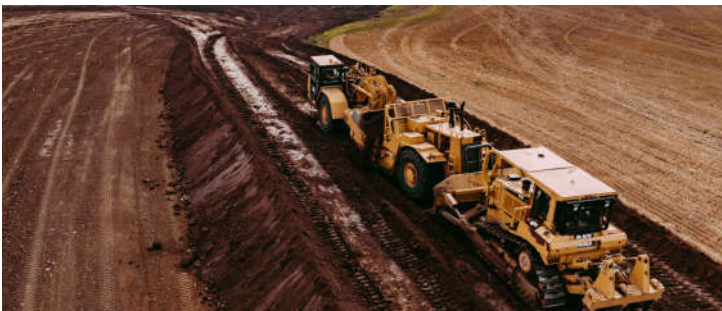
Improvement to sharp shoulders on Twp Rd 484
