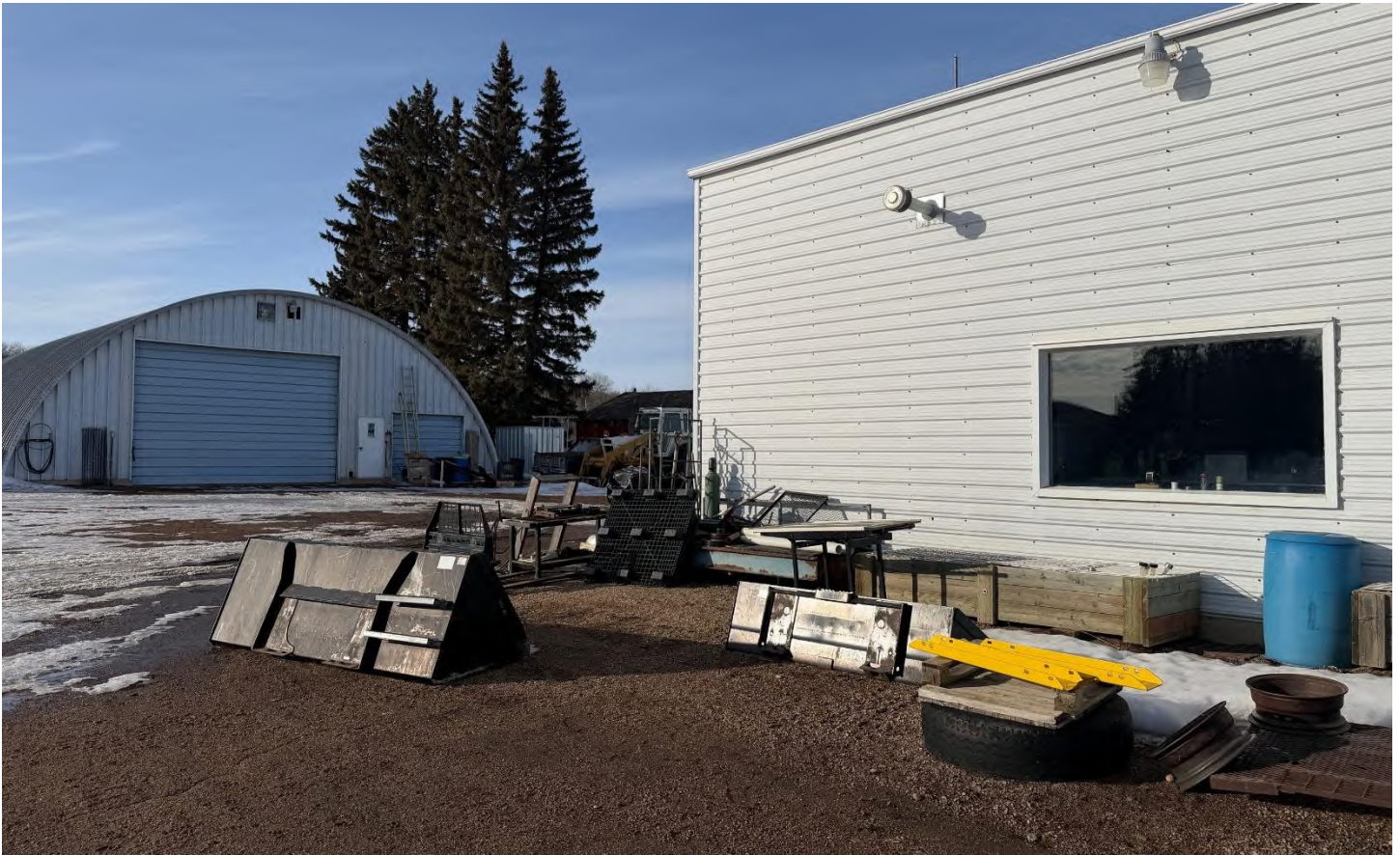
Water well under tire at shop within proposed Lot 1.
