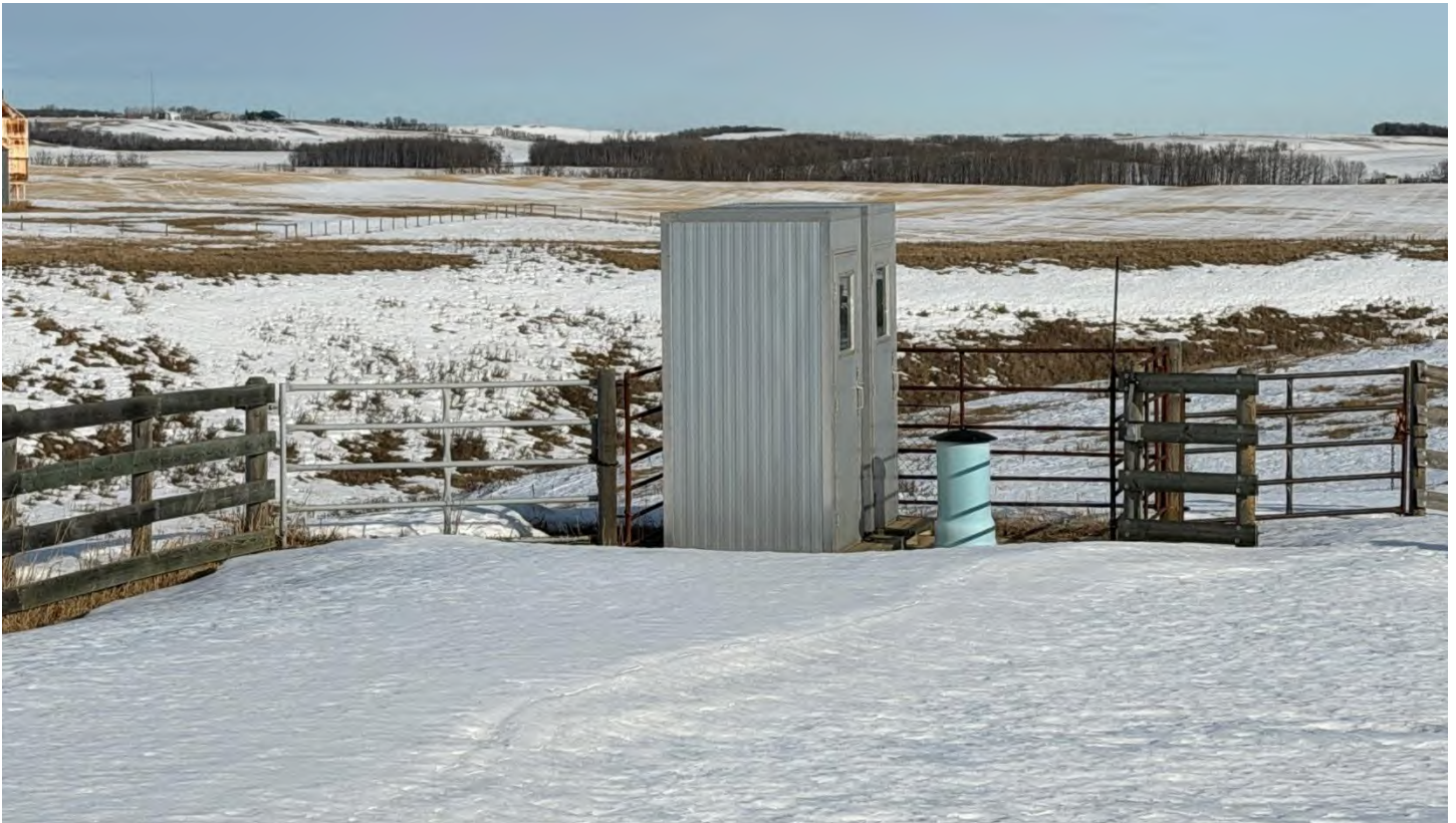
Another water well located in sheds within proposed Lot 1.
